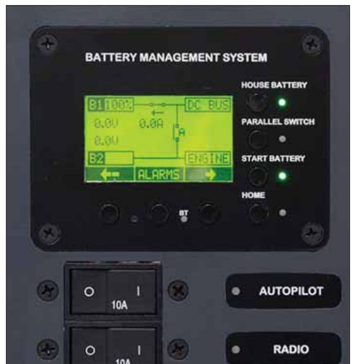
A lithium battery management and control system panel monitors the key parameters of the vessel battery system and provides remote control of the battery switches and charge system devices.
