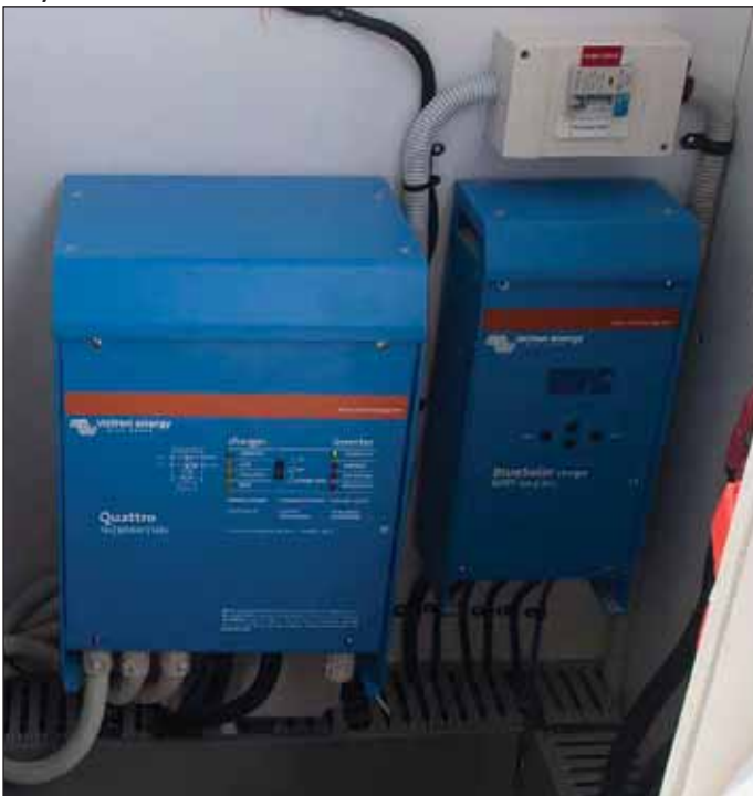
An inverter charger provides AC power when the generator is not running or when shore power is unavailable. The integral battery charger and adjacent solar panel regulator take care of battery charging.
