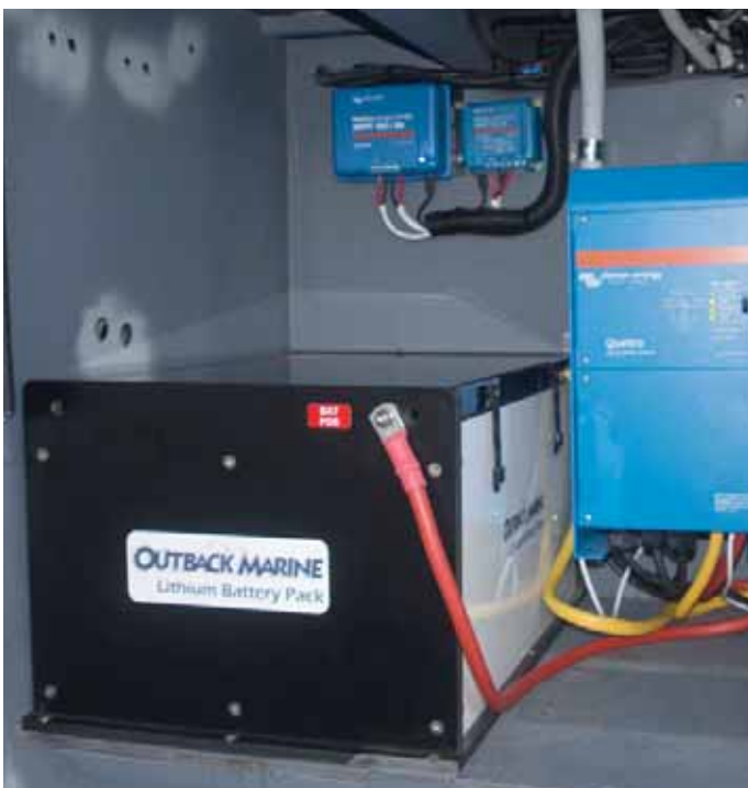
This installation shows a 24 volt 360 AH (8.5 Kwh) lithium battery installed in the same cabinet as other active electrical equipment. This installation is safe as lithium batteries do not produce a flammable gas when charging.
