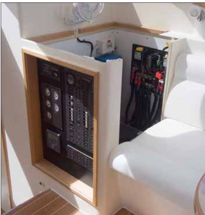
An electrical system cabinet on a Lightwave 38 sailing catamaran houses the electrical panels, DCD Board, Inverter Charger and Solar Regulator. The Lithium battery is under the settee to the right.
